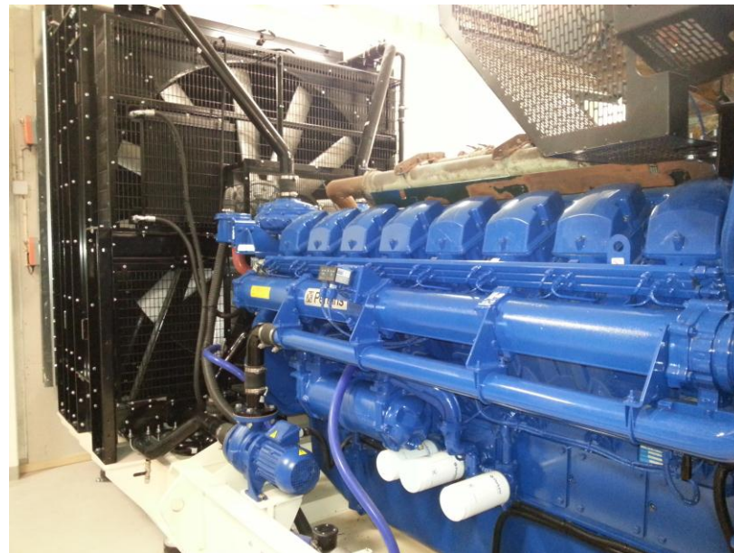
2,5 MVA power generators in N+1 configuration
