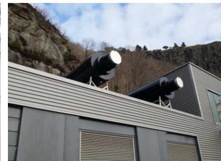
2,5 MVA power generators in N+1 configuration
